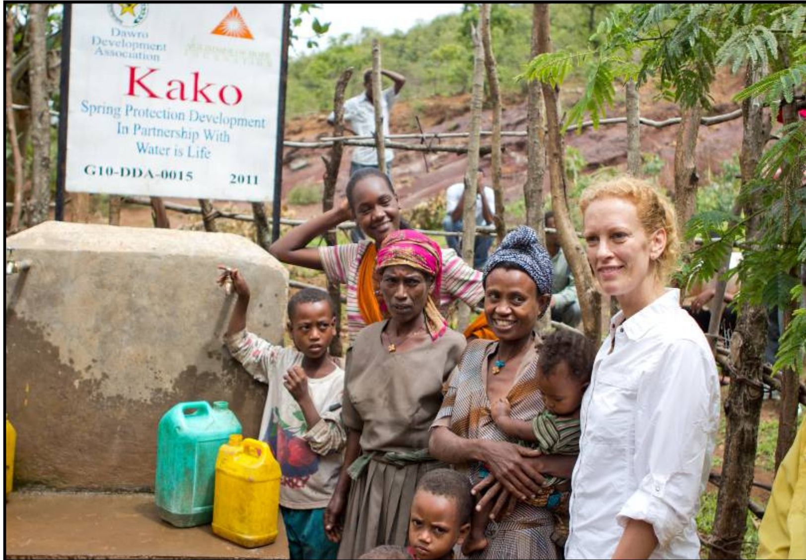
Water is Life - 2010 campaign Kako, Dawro– Spring Protection Development GPS Coordinates: lat/long: 7.137611, 37.150944
